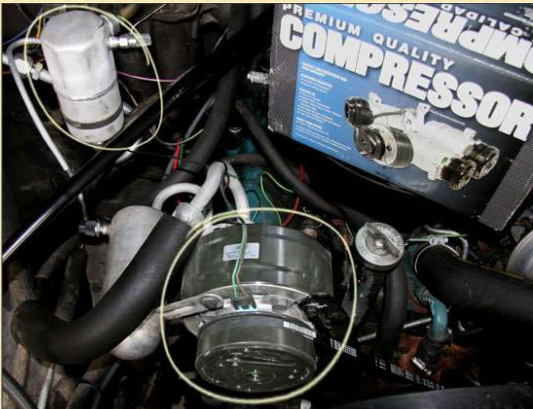
compressor & accumulator circled
